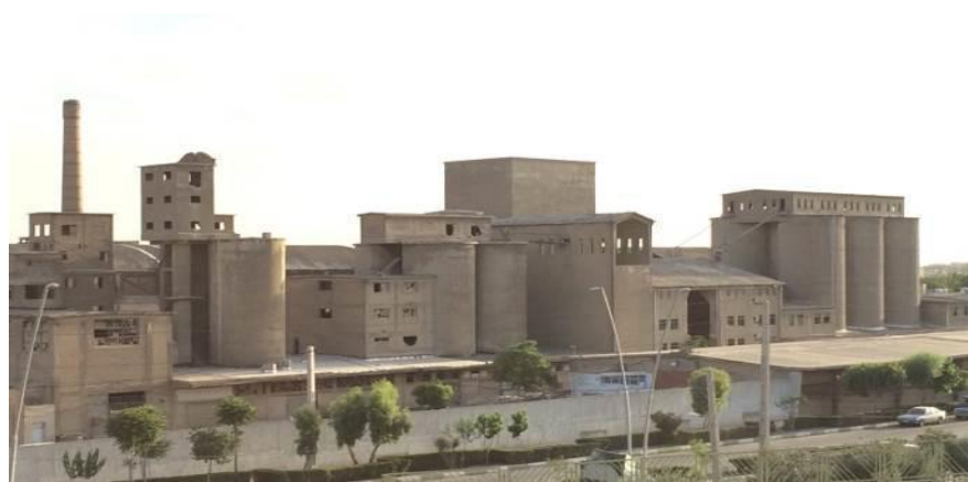
Fig 3. Silos located on the north side of the factory
