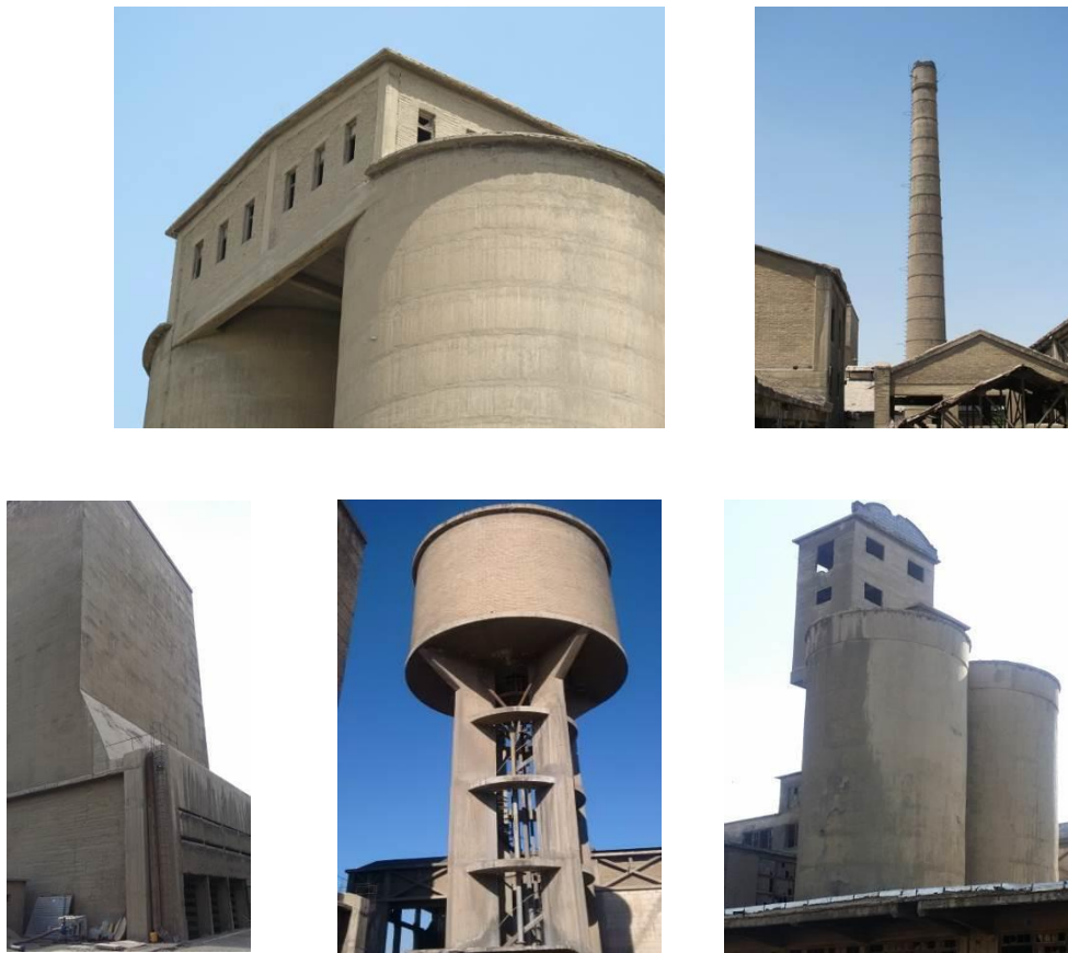
Fig 2. Current state of various components within the cement factory
